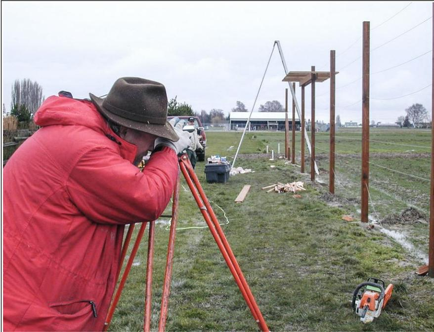
*Kristan using surveying equipment to lay out the espalier supports.*
